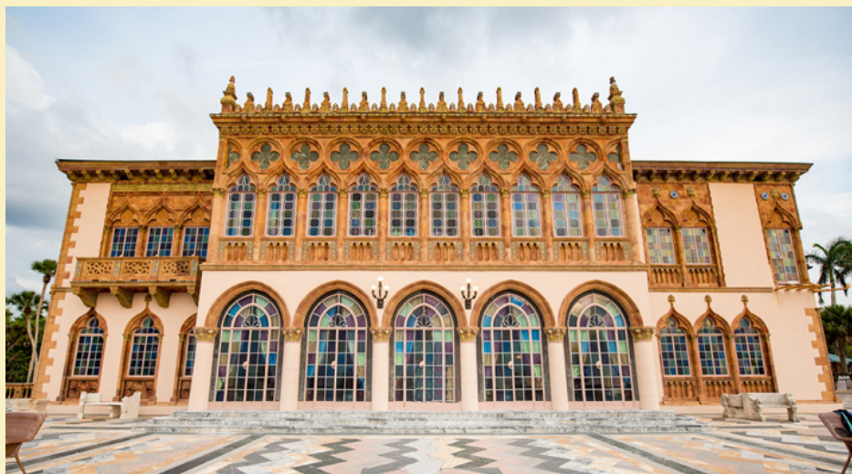
THE RINGLING RESIDENCE, CA' D'ZAN
