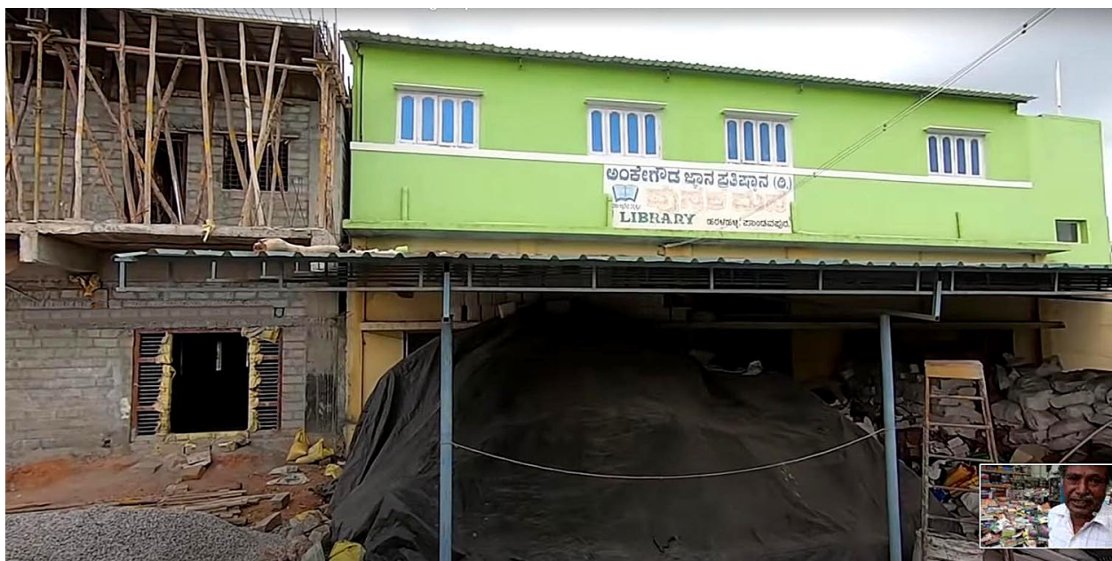
The House of Books. An addition is being constructed at the rear of the building (left). Books in large bags are piled under the shed-style roof.
